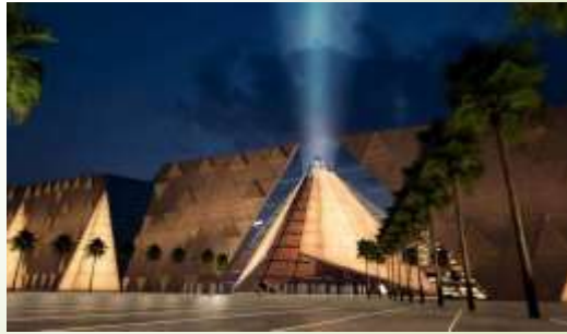
The new Grand Egyptian museum (under construction)
